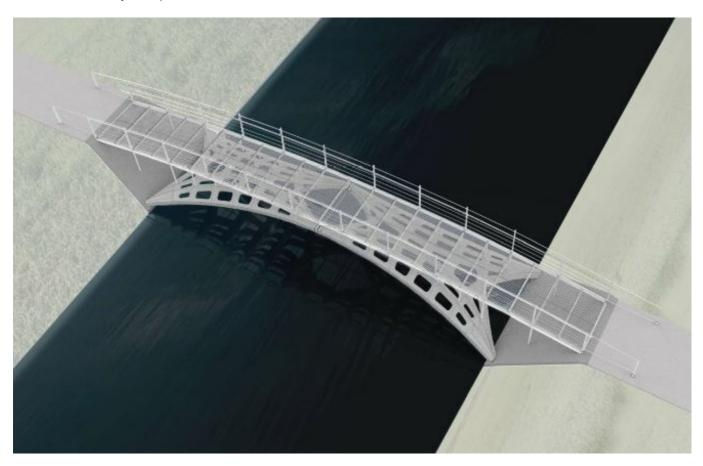
The concrete mixture which will be applied will be "green concrete", meaning made from recycled concrete. Thanks to its structure, building the bridge will require less material, thus reducing the addition of cement.
